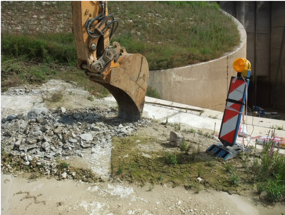
Bild 1: Schurf EB 1
